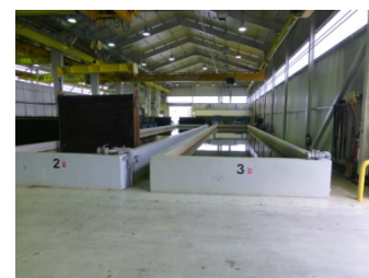
Storage Pits filled with water
